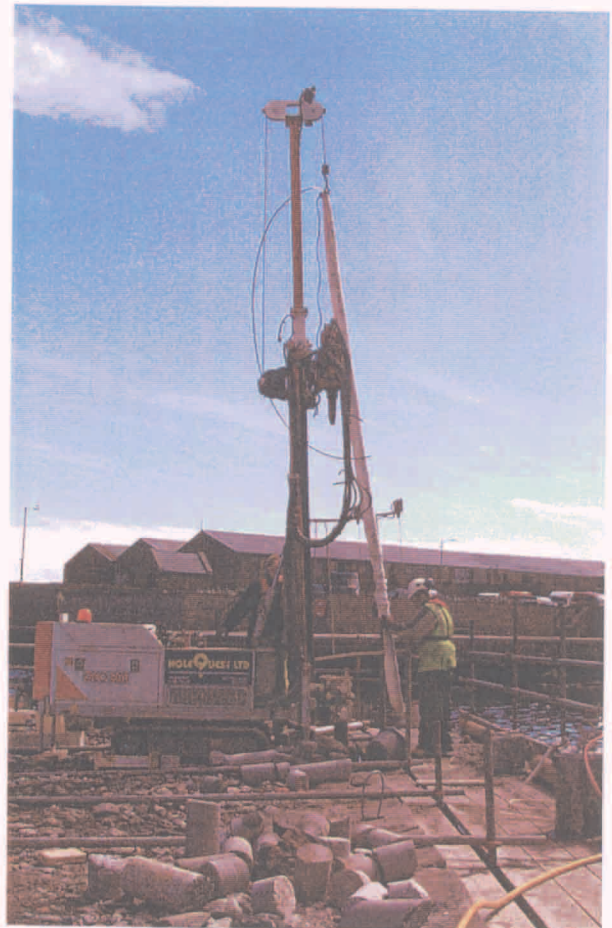
A mobile rig was employed firstly to core drill the anchor holes, then to temporarily install a metal tube hole lining, followed by the lifting and lowering of the Cintec anchor (above) and finally the removal of the temporary core lining prior to anchor injection.
