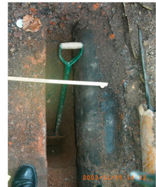
Fig 1. Excavations revealed a large gas main close to the north wall.
