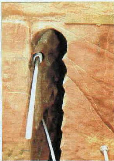
Below right: The 20 Cintec anchors were installed around the perimeter of the opening before extraction of the sandstone
