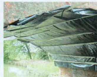
Temporary below arch protection during the installation process
