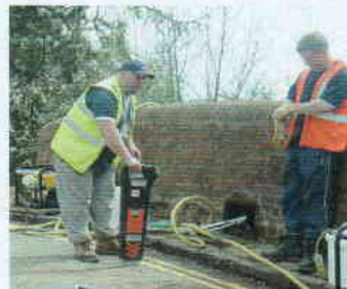
Checking for sub-surface services during bridge survey
