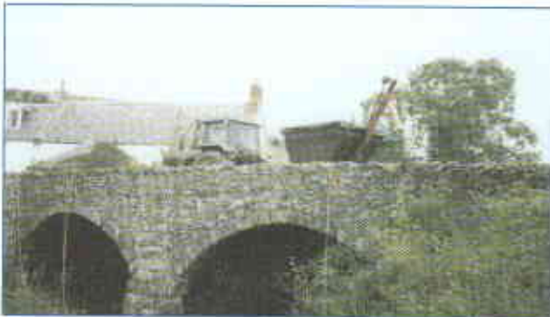
CLIFTON BRIDGE - SCOTTISH BORDERS
