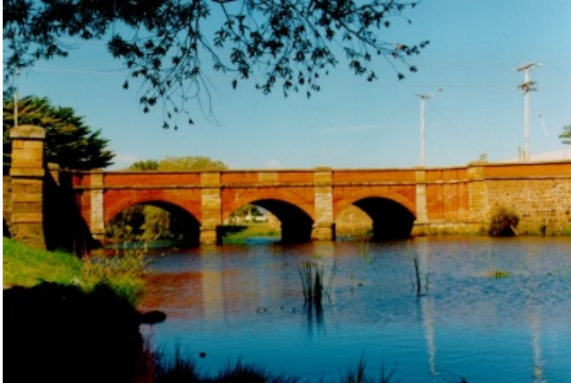
View from the west
