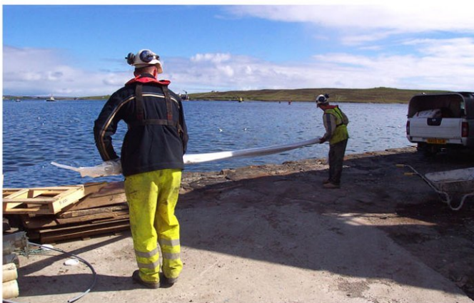
Cintec anchor being carried to the end of the quay ready for installation.
