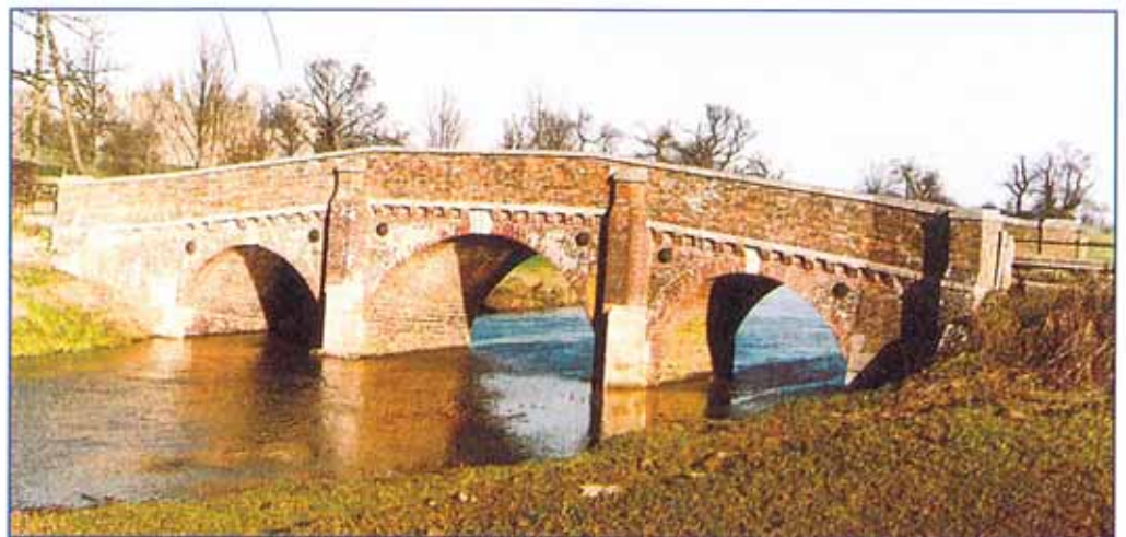
Bodiam bridge after completion with the castle behind the trees in the background.
