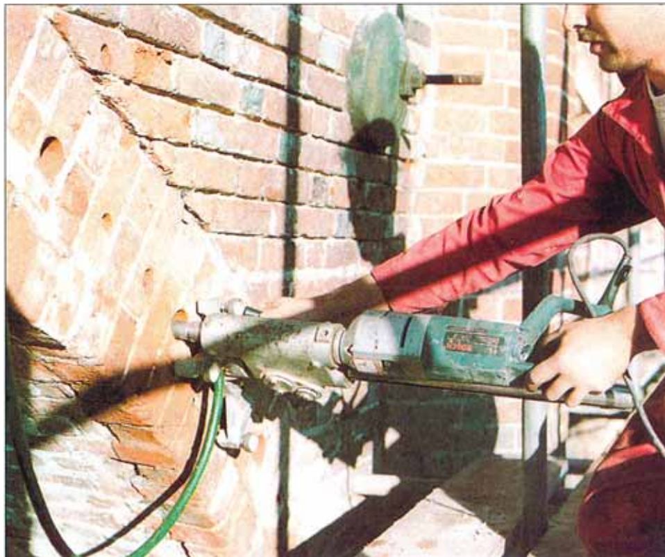
Core drilling holes for the anchors
