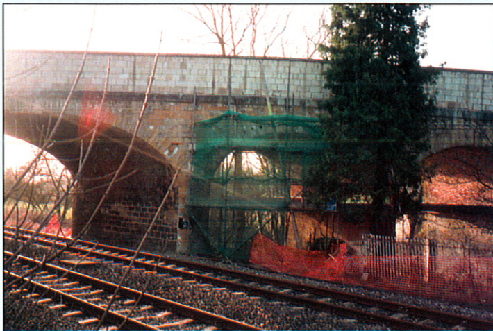
British Rail Bridge Stow-on-the-Wold
