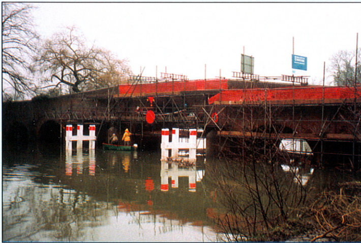
Historic Sonning Bridge at Reading
