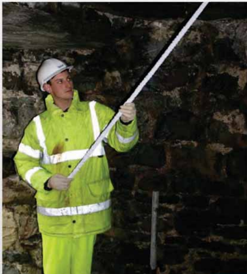
Installing anchor into diamond drilled hole to secure stones forming the floor/ceiling in the kitchen tower at Harlech
