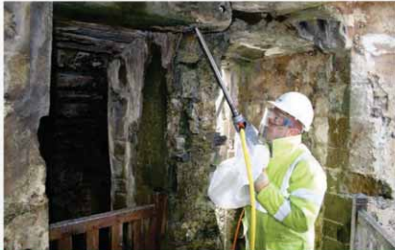
Diamond drilling to install anchors to secure a lintel over the doorway to the prison tower at Harlech
