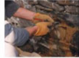
Insertion of 3m Cintec Anchor (left), and its inflation using cementitious grout, (above).
