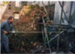
The process of diamond drilling (above), with the subsequent core samples produced, (left).
